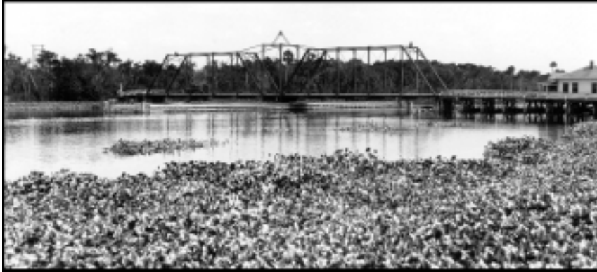
Figure 21. The first Monroe Bridge was operated by a hand-rotated crank turning draw mechanism (courtesy Jesse Beall, DeBary City Archives).
